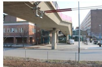
View from the lower level
