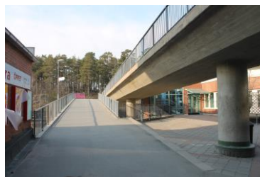
View from the opposite side
