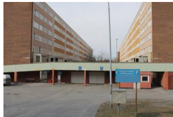
Example of short tunnels
